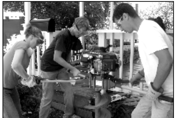
Marina Bronstein (left), Aaron Plave and Ariel Poliner use an auger to build Garcia’s ramp.
