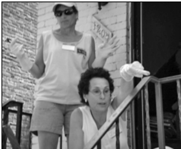
A fellow volunteer stands ready to help as Jill Kastner, Jason's mother, works on a railing at Mitzvah Project house.
