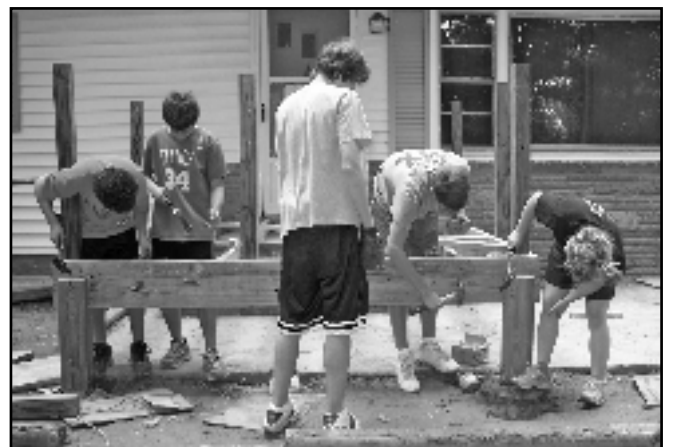
Maria Mae Taylor’s ramp takes shape as ramp campers hammer away.
